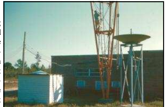
Behind the building were 2 microwave dishes. The one on the white building is the studio feed and the other is the Telco feed for the NBC programs. Relay dishes are not allowed to point up now due to satellites. There was only one satellite in 1955, the moon! The first man made satellite was launched 2 years later, October 4, 1957.
