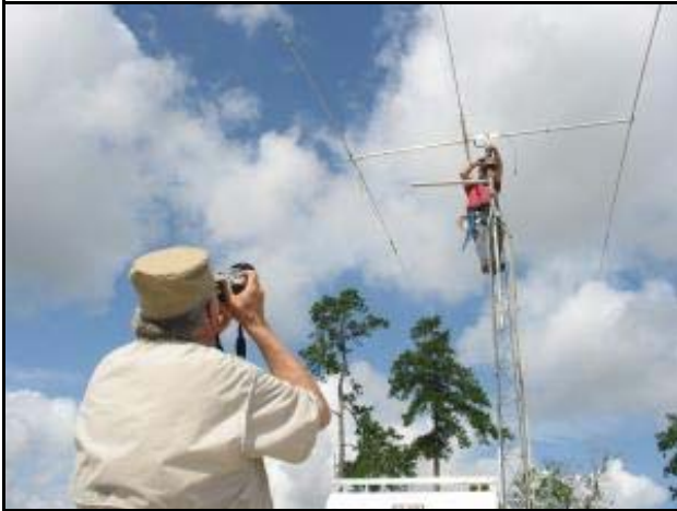
John McCoy, K4KBB , taking picture of Bernie Nobles, WA4MOK , installing TA-33 Jr. on the tower.
