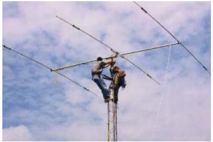
Pat Sutton, KD4NNA, and Bernie Nobles, WA4MOK, putting the finishing touches on the Mosley beam.
